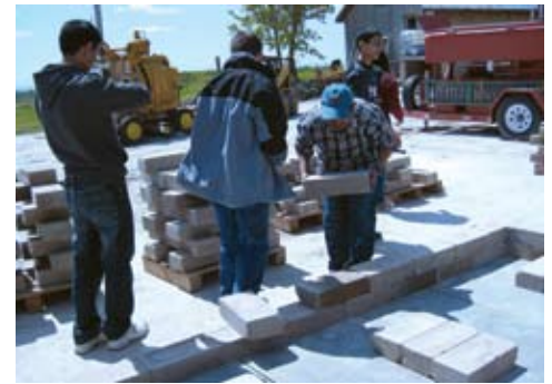
Students do a "dry" build, Earthblock machine in background
